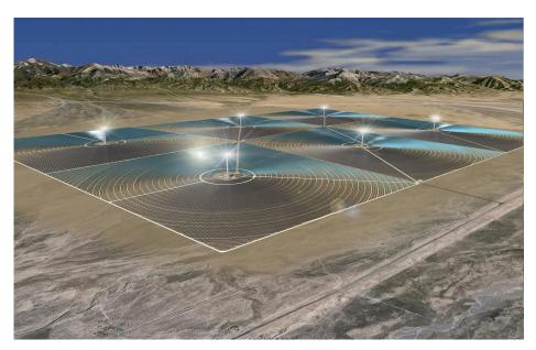
The first phase of the Qinghai Delingha Solar Thermal Power Generation Project will use BrightSource's proven solar tower technology to produce clean, reliable solar electricity to more than 452,000 residences. Located in the Qinghai province in northwest China, the Delingha project is planned for six 135 MW CSP tower plants. The first phase will include two 135 MW solar thermal plants with up to 3.5 hours of thermal energy storage.
